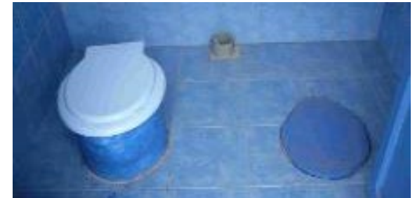
Poor ventilation design
